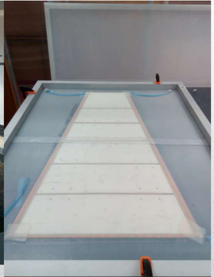
Frame gluing under vacuum
